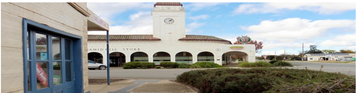
Pyramid Co-Op Building Built c.1935
